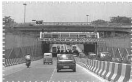
A passage below a road .....
