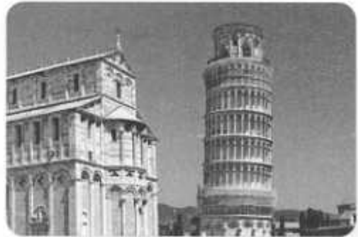
A tilted tower that is part of a church
